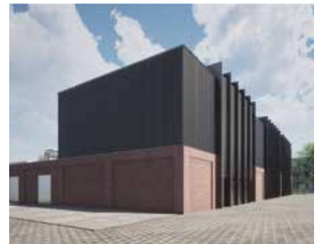
Transformatorstation IJburg, Amsterdam
